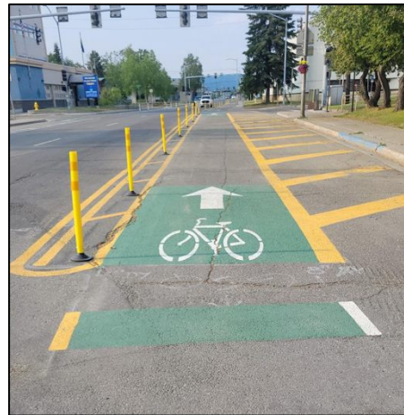
Fairbanks Pilot Bike Lanes Project – photo by Evee Rynish
